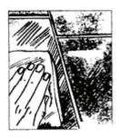
5. After grout has set hard to the touch, clean surface of slate and along grout line by rubbing briskly with a clean piece of cloth.
