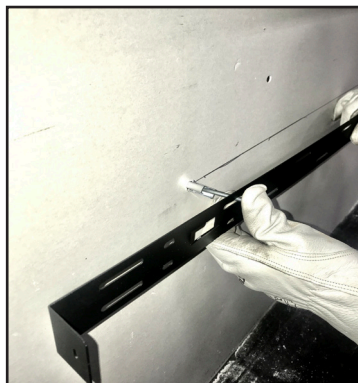
Figure 4.5 Installing Anchors in Hollow Wall
