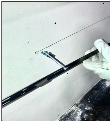
Figure 4.4 Toggle Bolt Installation through Mounting Bracket
