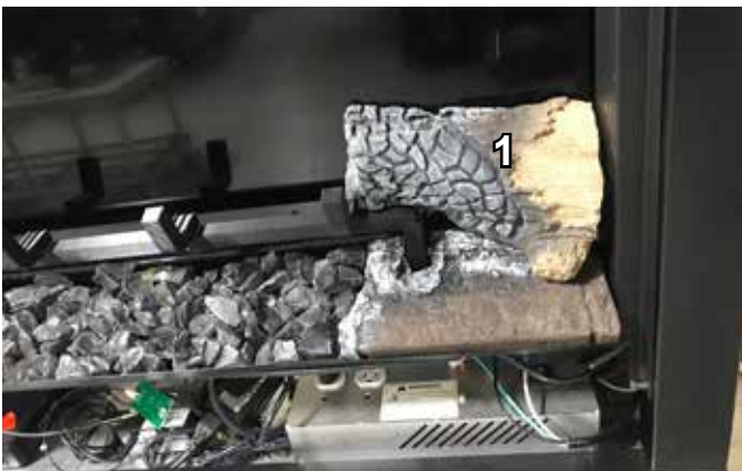
Figure 4.21 Install Log #1
