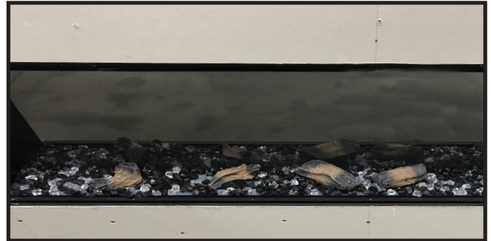
Figure 4.10 Media and Small Logs Installation
