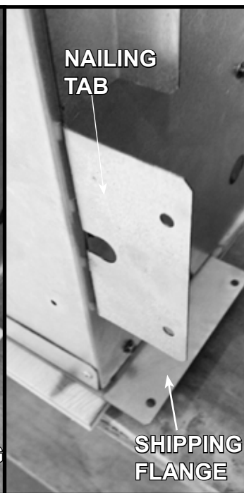
Figure 6.7 Nailing Tabs Installation Position
