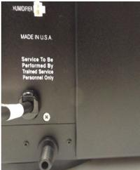
**NOTE:** Wine Guardian unit has an internal trap. Do not double trap piping. Failure to comply may lead to water leaks and possible water damage to surrounding mounting area. Install drain line with a 1/4 inch per linear foot (1.25 cm/linear meter) of pitch.
