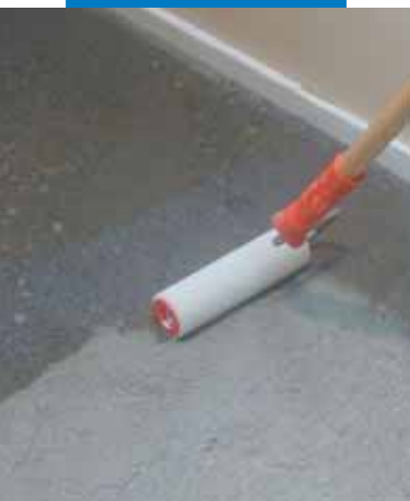
Applying Primer G with a roller
