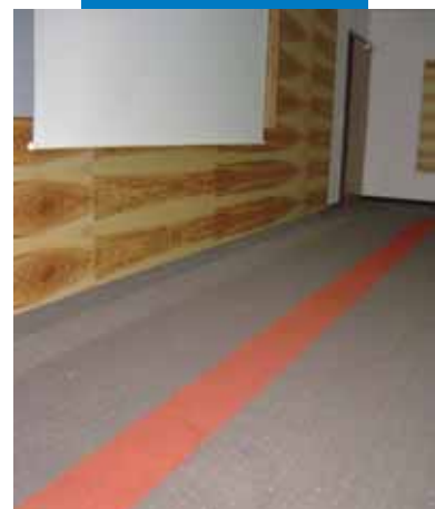
Example of Primer G applied before spreading on Ultraplan Eco and Rollcoll adhesive, used to bond carpet in a hotel room - Villa Hotel Castellani - Austria
