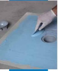
Impregnating Drain Vertical fabric with Mapelastic<sup>®</sup> AquaDefense
