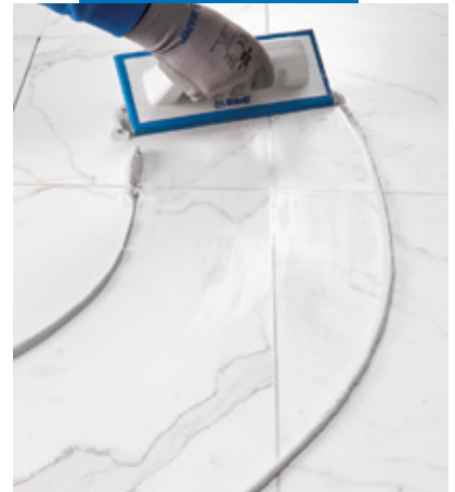
Spreading Ultracolor Plus on marble-effect porcelain floor tiles with a rubber trowel
