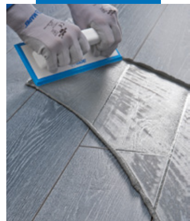
Spreading Ultracolor Plus on wood-effect porcelain floor tiles with a rubber trowel
