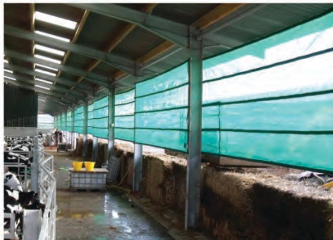
Fig 9 Windbreaks fitted inside and outside
