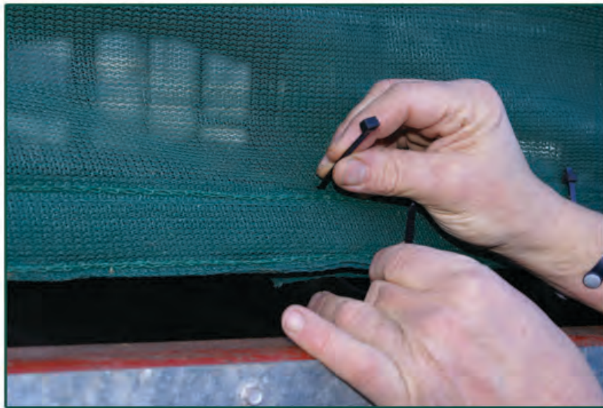
Fig 6 Fixing cable ties
