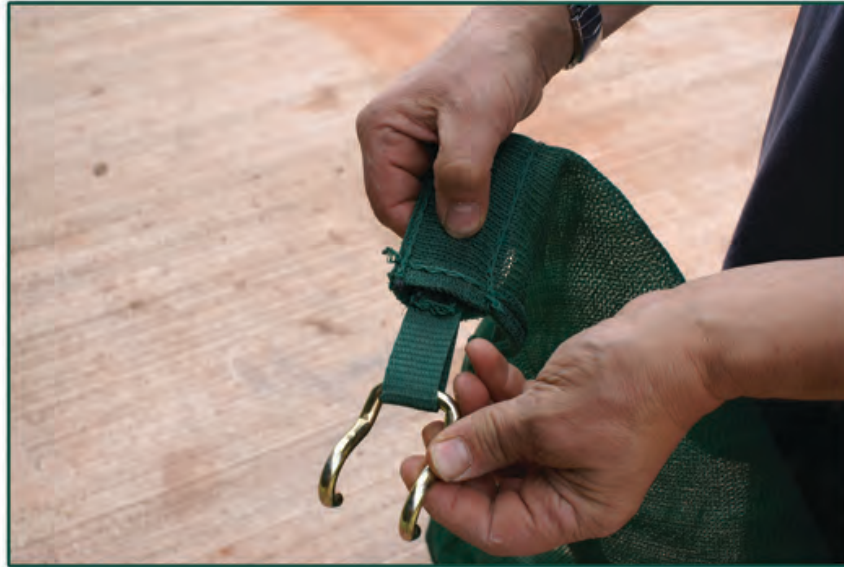
Fig 1 Fitting a loop hook.
