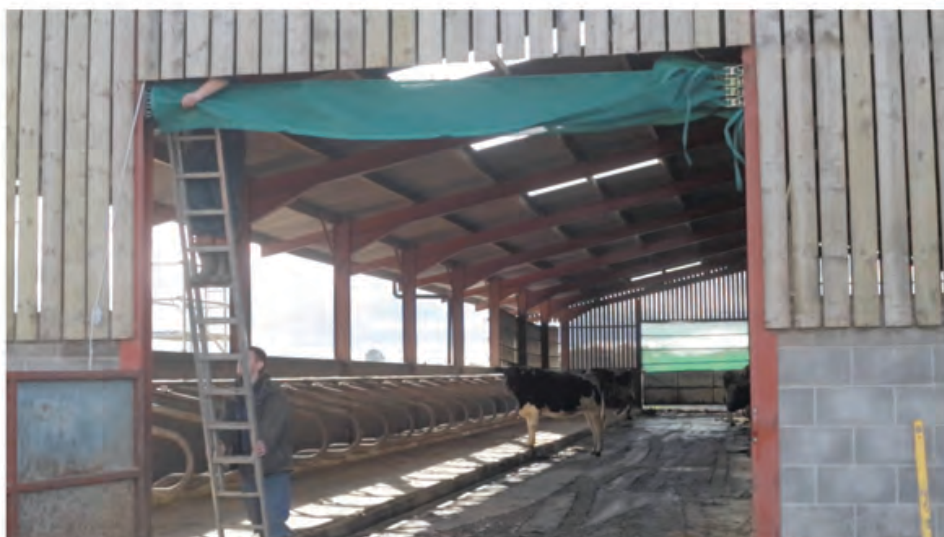
Fig 9 Attaching Econoblind to top fixed trolleys
