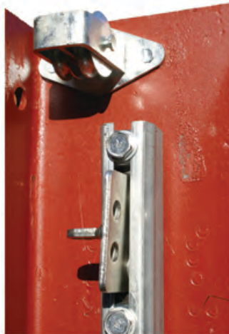
Fig 5 Pulley above track
