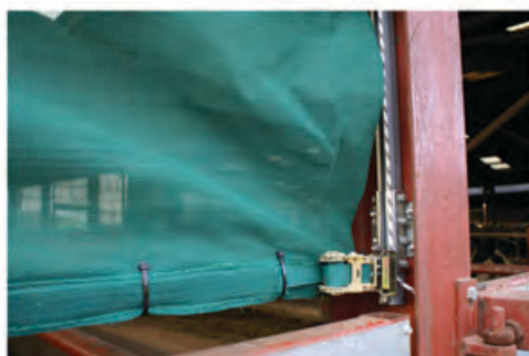
Fig 14 Trimmed cable ties
