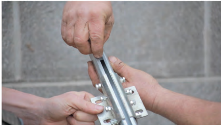
Fig 2 Joiner/fixing plate 12cm from top
