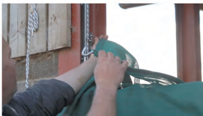
Fig 7 Attaching the windbreak to the trolleys
