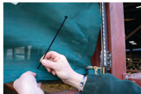
Fig 12 Cable tie pushed through
