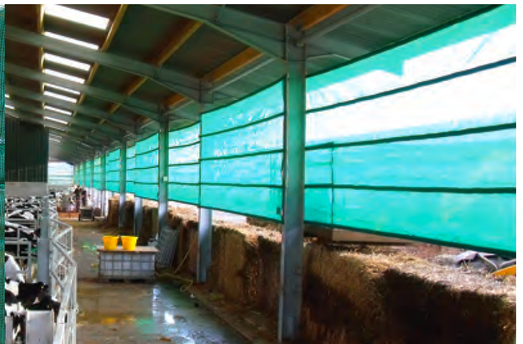
Fig 9. Windbreaks fitted inside and outside
