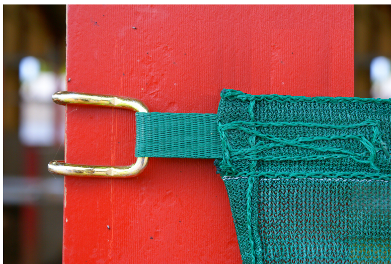
Fig2. Loop hook attached to H-beam
