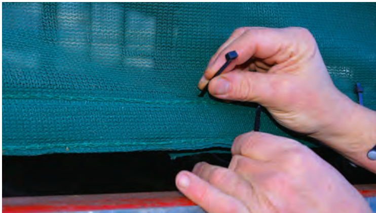
Fig 6. Fixing cable ties
