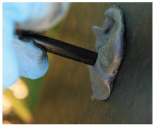
**Step 5:** Apply epoxy to fill the hole that the cord is running through. Ensure enough slack is in the cord so you can position the kit in the center of the planter. Wait at least 1.5 hours for the epoxy to harden. Do not move the cord during this time.
