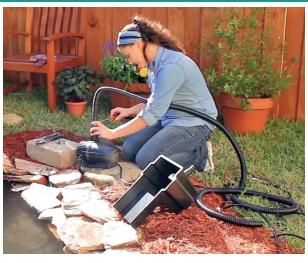
**Step 2:** When you are happy with the location of the waterfall, connect the tubing to the pump.
