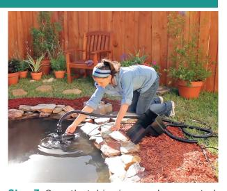
**Step 3:** Once the tubing is securely connected, place the pump in the pond.
