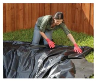
**Step 4:** Lay the liner. There should be at least a 10-12 in. overhang. If roots and/or debris are present, line the bottom with old carpet or sand to protect the liner from punctures.
