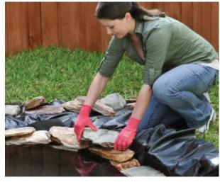
**Step 10:** While the pond is filling, secure the liner with stones. Add a ledge of decorative rocks around the perimeter to hide the liner edge. The ledge can be a couple of inches deep.
