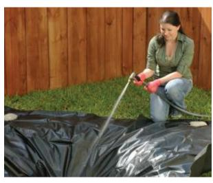
**Step 5:** Begin filling the pond. Adjust the liner edges, smoothing any wrinkles as it fills. Stop filling halfway.
