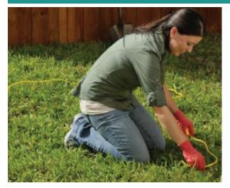
**Step 1:** Start by using a piece of string or rope to mark the shape and location of the pond. This pond is approximately 3 ft. x 6 ft., with a depth of 1.5 ft.
