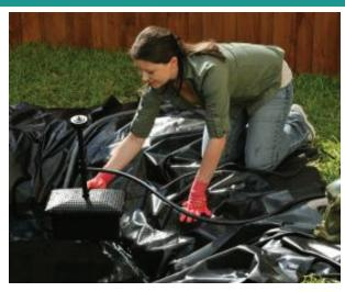
**Step 8:** Place the Complete Filter Kit with Pump assembly in the center of your pond and continue filling the pond with water.
