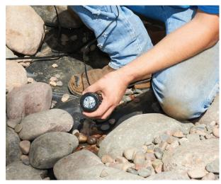
**Step 4:** Add pump with assembled nozzle kit and lights to pond. Position the lighting and run the power cord to the outside of the pond; cover cords with rock.
