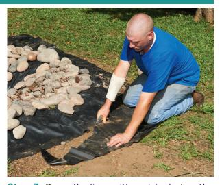
**Step 3:** Cover the liner with rock including the 10-12 in. around the perimeter; leave a small area void of rock to run the cords outside the pond. Trim away excess liner.
