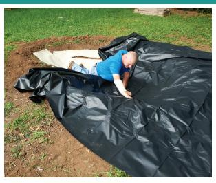
**Step 2:** Cover the entire area with the liner. The liner should extend over the sides of the pond by 10-12 in.
