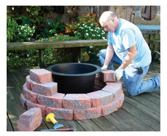
**Step 2:** Begin building the next tier of the pond wall. Each block has a "lip" located on the back of the stone. This lip creates a locking effect. When placing the lip down, make sure it is centered over the gap of the bottom tier. Repeat step three for the third and fourth tiers.
