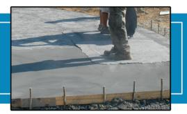
Liquid Release is a bubble gum scented colorless liquid release agent specially formulated as a bond-breaker between freshly poured concrete and decorative tools such as stamp mats, texture skins, stencils, etc. It creates a lubricating barrier that extends the life of the texturing tools by decreasing the friction between the concrete and the tools. Liquid Release evaporates leaving no residue behind, meaning less clean-up and labor cost. This
