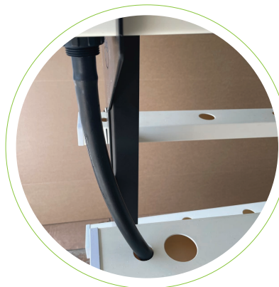
CHANNEL OUTLET Fitted and in place.
