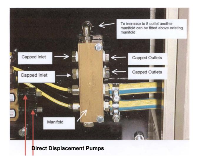
This system can be increased to a 4 nozzle system with existing manifold. Requires 2 extra displacement pumps added to bridge above existing displacement pumps.
