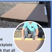
sides are level. Adjust the ground/blocks as needed.
