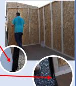
Push the wall in against the floor the whole way across. Fasten the pre-started screws in the wall into the floor.
