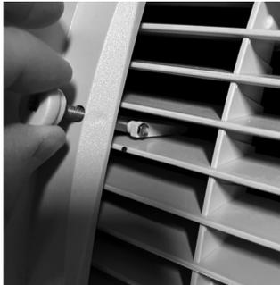
5. Tighten nut loosely to secure in place but leave room to install side frame.
