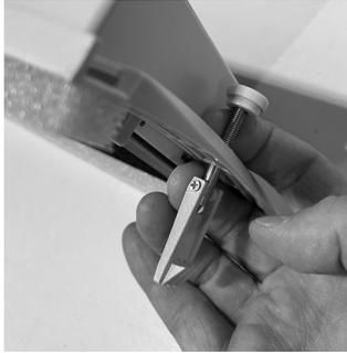
2. Install the Optional Attachment Clamp and leave nut loose to allow for center frame attachment to the PTAC unit.
