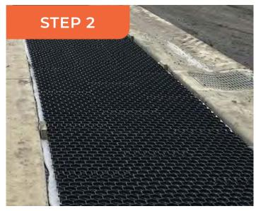
If the base is a reactive soil or sand, lay a geofabric over the leveled base before installing an aggregate drainable road base.
