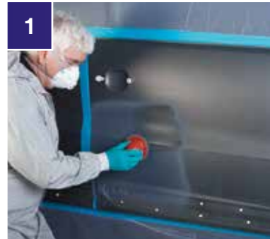
1 Apply 3M™ Dry Guide Coat to primed surface.
