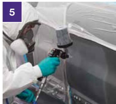
5 Apply high build primer to repair area using 3M™ Accuspray Gun and 1.8mm nozzle.
