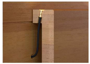
Some of the fibers may be installed on the sauna benches or backrests. The picture shows the installation of the fiber from the backrest upwards. To get the best lighting result, it is a good idea to drill the installation holes so that the fiber is about 10-15° away from the wall.
