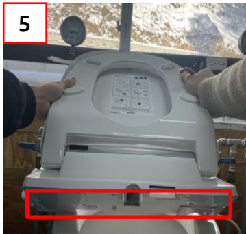
5 Push the bidet back so that the bottom of the bidet is visible. (Angle: 45 degrees)
