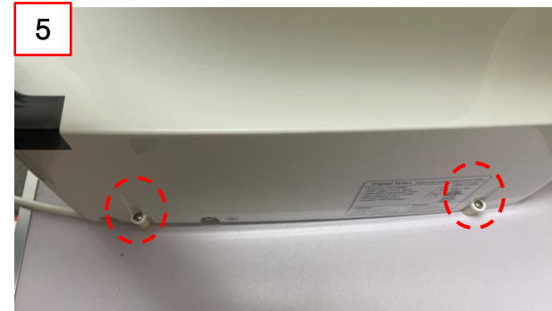
⑤ Screw the two screws at the back of the bidet
