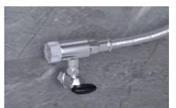
1 Disconnect the strainer filter from the hose and valve.
