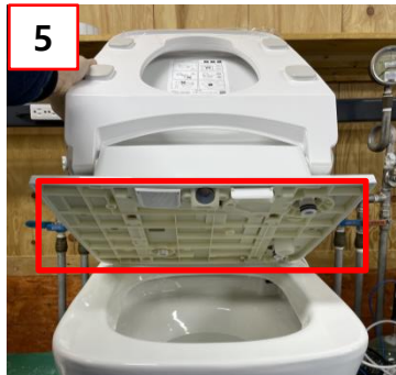
Push the bidet back so that the bottom of the bidet is visible. (Angle: 45 degrees)
