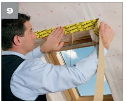
• Finally seal the overlaps using Sicrall 60
