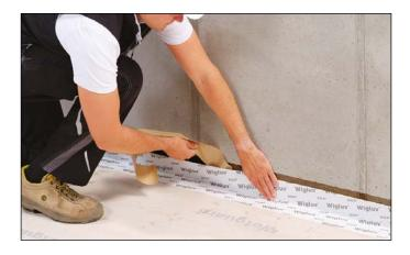
Seal transitions to mineral substrates (concrete, cement-bonded particleboard) with Wigluv 100 or wider:
