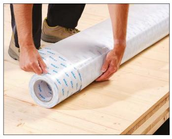
Remove larger backing and adhere the first 1-2 ft while ensuring straight application
