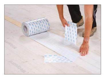
Bond element connecting joints (spline joint) with Wetguard 15" or wider
