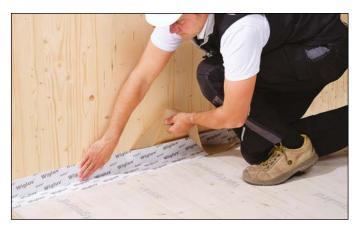
Seal transitions to timber materials with Wigluv 4" or wider or Wetguard 15":
