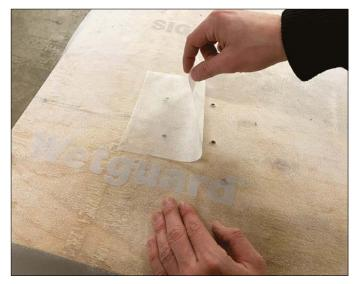
Apply a piece of Wetguard 200 SA or Wigluv to face of Wetguard 200 SA field membrane, centered over damage, and extending past
