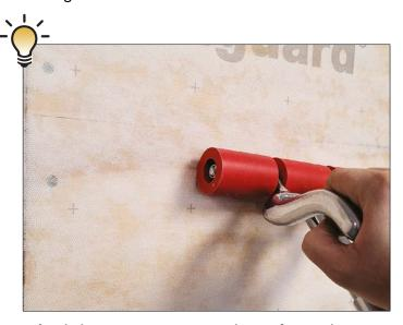
Apply heavy pressure to entire surface using a heavy steel roller to obtain optimal adhesion
