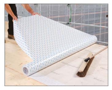
Gradually remove backing while pressing on using a broom, squeegee, or J-Roller
