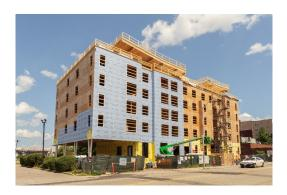
SIGA's Majvest® 500 SA (left) is a vapour permeable self-adhering water-resistive barrier and air barrier membrane for both commercial and residential buildings, such as the multi-level wood frame building shown on the right.
