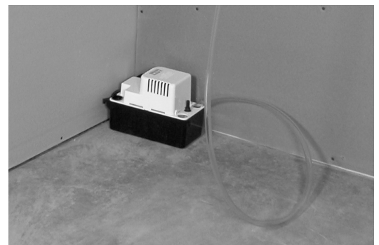
figure 9.2 Use a condensate pump if you don't have access to a drain.
