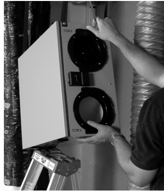
figure 6.2 Pull on the middle strap and gently push upward on the unit. Then repeat procedure on other side.
