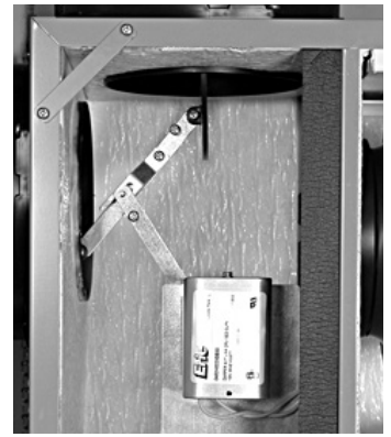
figure 8.3 - Motorized Damper Assembly
