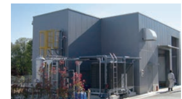
The Tokyo Plant water treatment facility
