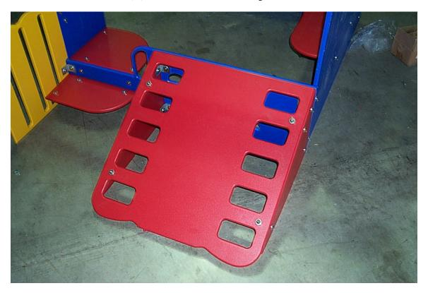
15. Install 8 corner brackets to the 8 remaining holes in the back panel (A) and the front entry panel (D). These holes are located along the top edge and will be used for the roof panels (P).
