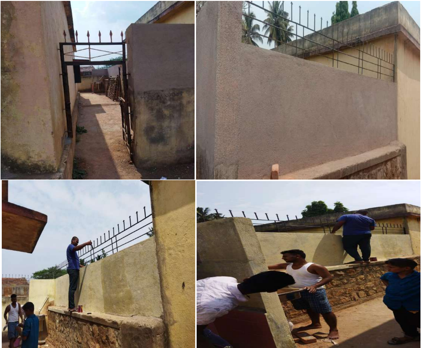
Figure : Toilets Renovation in progress at murgod,belgaum,india.
