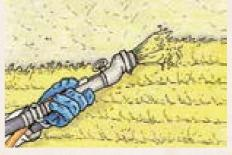
5. Wet the surface and apply a second coat of SANACOLOR 2000 plaster in a thickness of about 5 mm
