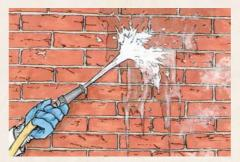
Wash the wall surface of the wall to remove the debris and residual salts. Wet new walls thoroughly.
