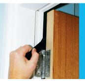
Insert Door Attachment into the door jamb, with hinges facing towards you, as pictured.
