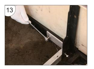
11. Secure the connection between the M8 x 30mm countersunk head screws and the aluminum alloy plate with a cross screwdriver and a 14mm wrench.
