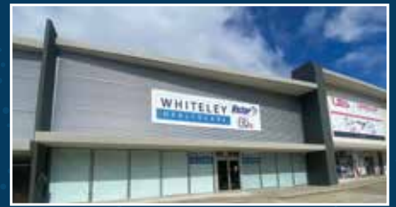
WA Store & Warehouse
