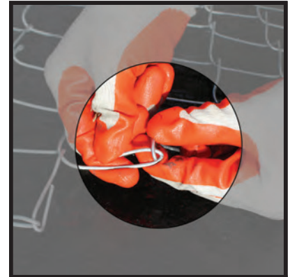
Figure 6-C Pinch Knuckles Closed
