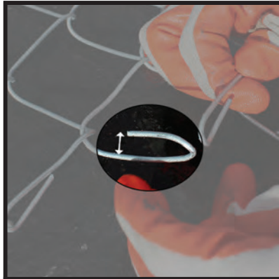
Figure 6-A Open Knuckle Example
