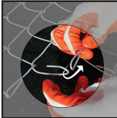
Figure 6-B Knuckle Nesting Example
