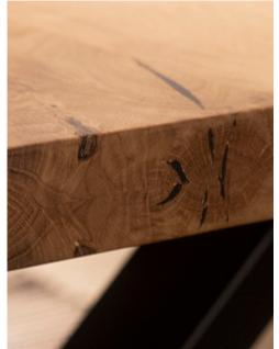
Example of fill-ings of cams and cracks with a black paste. The paste prevents dirt and grime from accumulating in the cracks.
