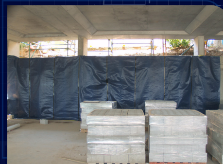
RETAINING WALL AT NSW RUGBY CENTRE OF EXCELLENCE
