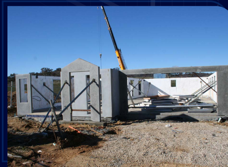
TILT PANEL CONSTRUCTION
