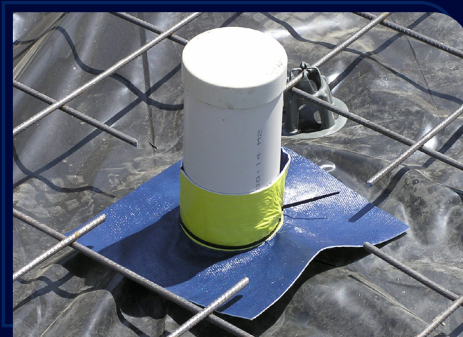
PROTECTION OF PENETRATIONS
