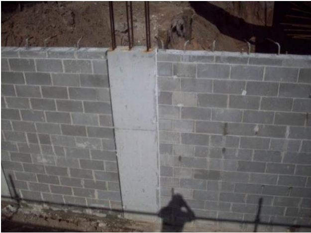
Figure 44 NOVITHOR Flexi-Gel in control joint.
