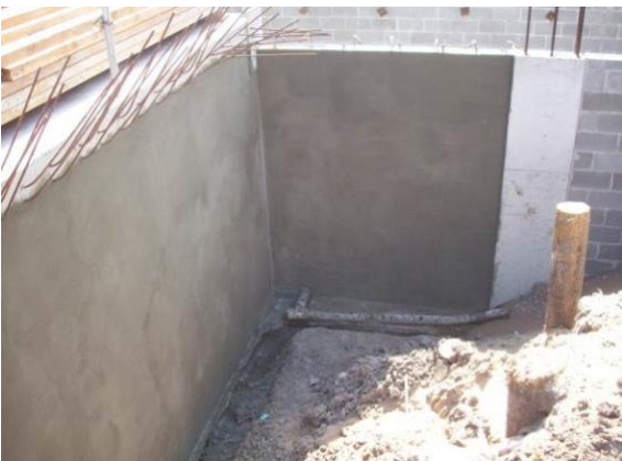
Figure 5 Second coat applied after the first coat application is touch dry. The final minimum thickness must be 4 mm.
