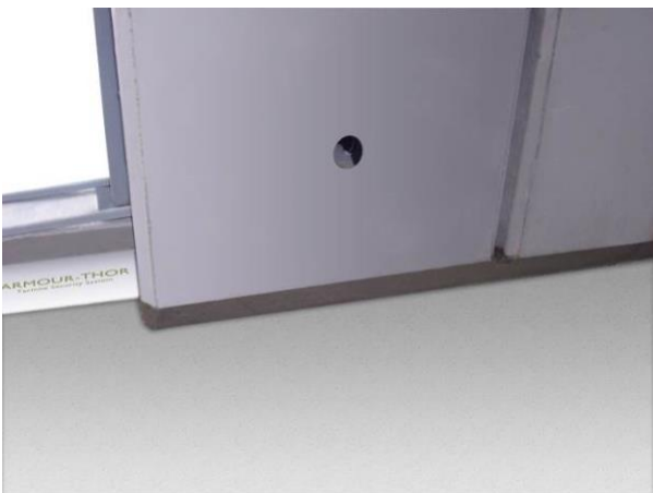
Figure 26 NOVITHOR Cementitious Parge positioned below tilt panel and on concrete slab.
