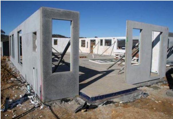
Figure 24 Tilt panel slab placed by builder.
