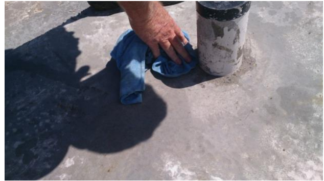
Figure 18 Wipe pipe and surrounding slab clean using a wet rag.
