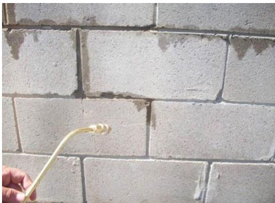
Figure 37 NOVITHOR Resin being applied to mortar joints in retaining wall.
