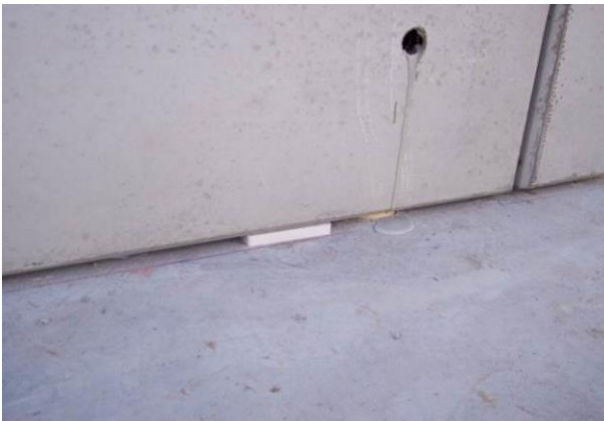
Figure 25 Tilt slab panel to be grouted with NOVITHOR Cementitious Parge.
