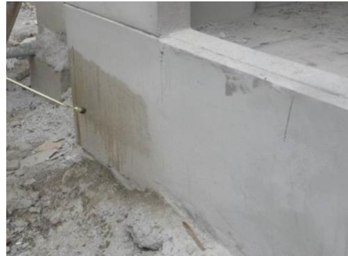
Figure 38 NOVITHOR Resin applied to rendered wall.
