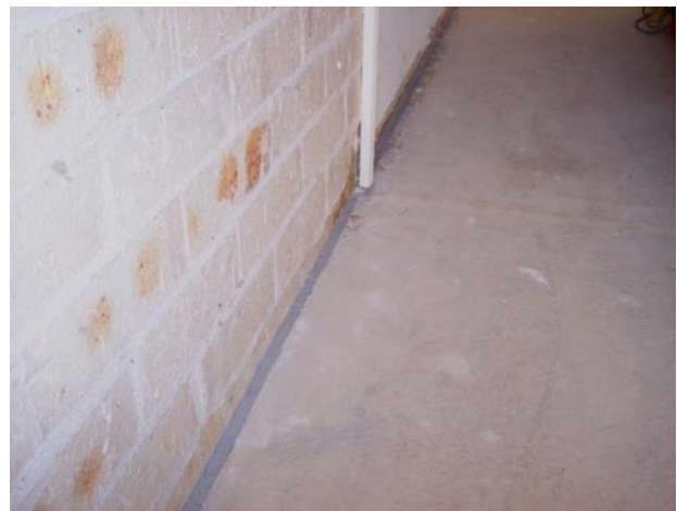
Figure 47 NOVITHOR Flexi-Gel between footing and garage floor in-fill slab.
