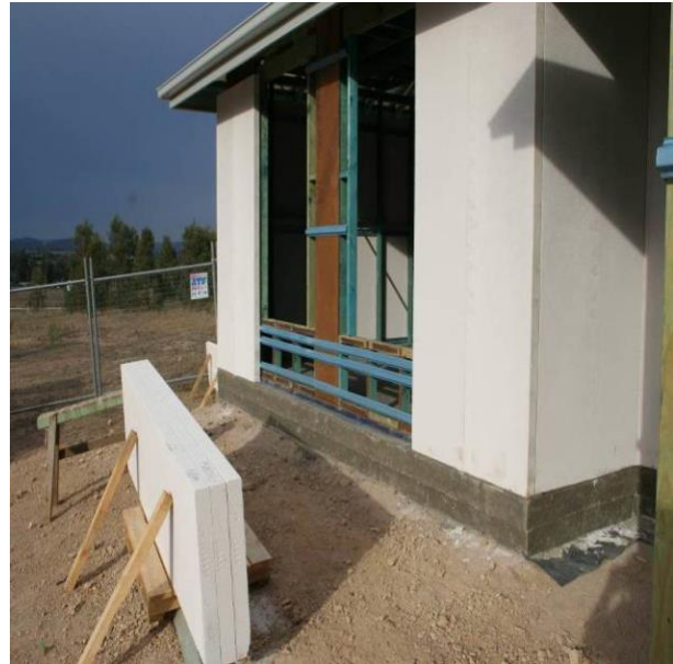
Figure 27 NOVITHOR Cementitious Parge applied over CSL Hebel and concrete slab edge.
