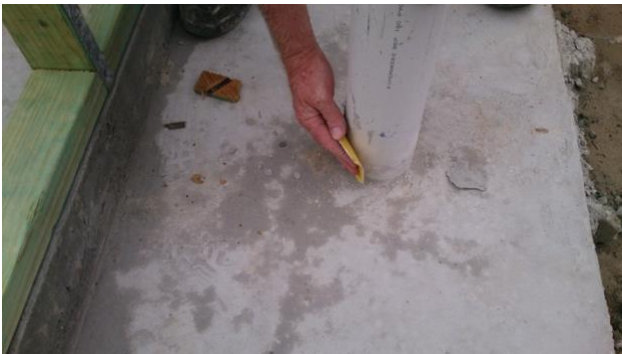
Figure 16 Clean any excess concrete from the edge of the pipe using coarse sandpaper.
