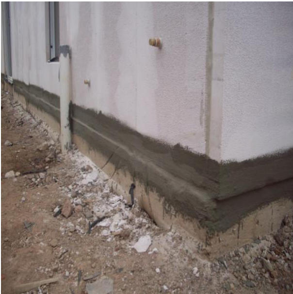
Figure 29 NOVITHOR Cementitious Parge applied over CSR Hebel and concrete slab edge.
