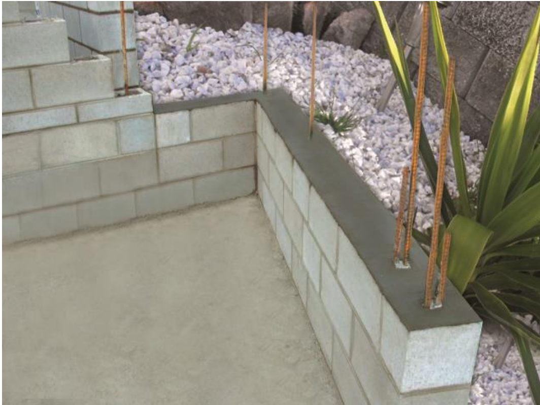
Figure 32 NOVITHOR Cementitious Parge capping RC block wall
