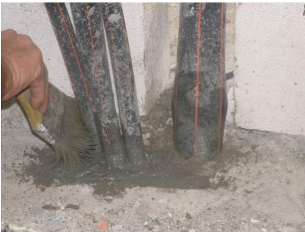
Figure 19 Apply NOVITHOR Cementitious Pargolite with soft bristled brush.
