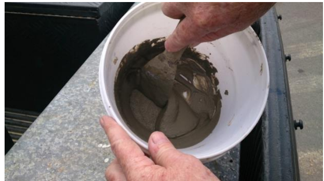
Figure 19 mix TPC Powder and TPC Liquid to a wet consistency to flow into the recess around the pipe.
