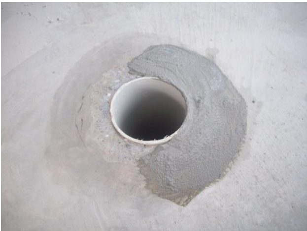
Figures 20H – 20I Apply the NOVITHOR Cementitious Parge so as to fill the trench and ensure it is flush against the exposed walls of the pipe penetration.
