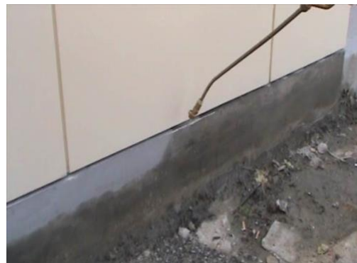
Figure 40 Resin being applied to rendered wall.
