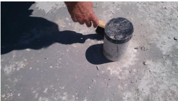
Figure 17 Brush dirt and loose concrete from the base of the pipe and surrounding slab area.
