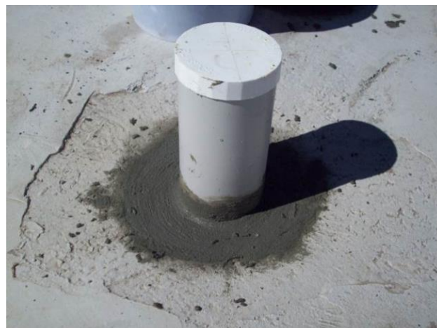
Figure 17 Brush dirt and loose concrete from the base of the pipe and surrounding slab area.
