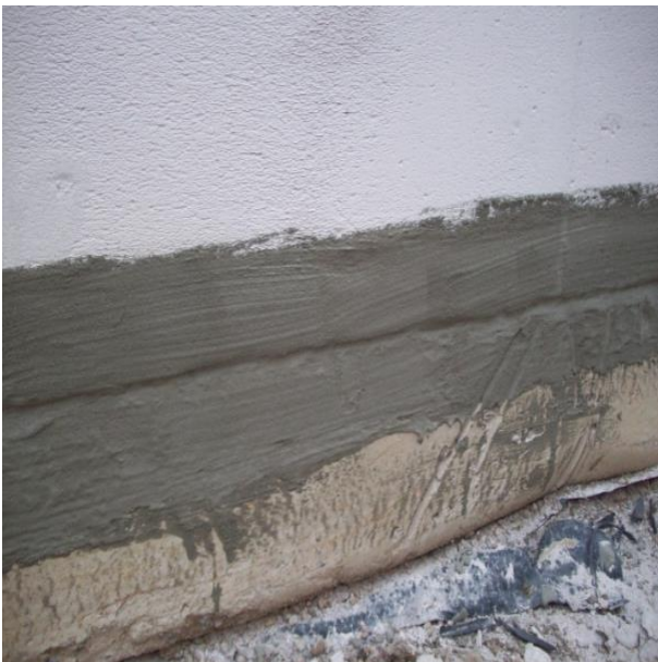
Figure 30 NOVITHOR Cementitious Parge applied over CSR Hebel and concrete slab edge.
