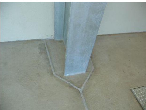
Figure 50 NOVITHOR Flexi-Gel around column.
