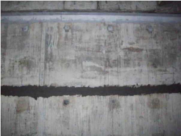
Figure 9 NOVITHOR Cementitious Parge over cold joint in RC retaining wall.
