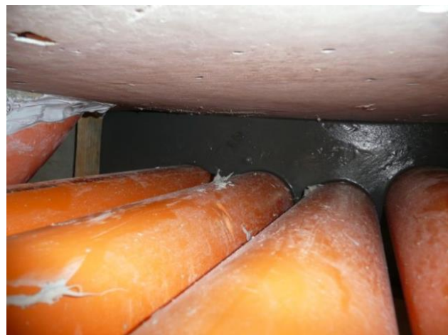
Figure 22 Ensure joint between pipe and concrete is fully covered. Cover cold joint between slab and RC column.
