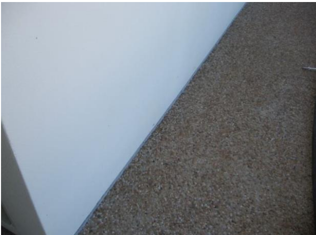
Figure 45 NOVITHOR Flexi-Gel in joint between wall and pavement/ concrete apron.
