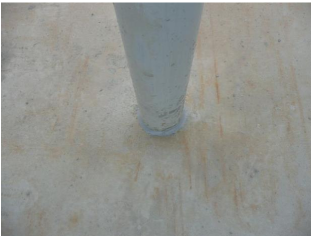
Figure 49 NOVITHOR Flexi-Gel around core drilled pipe.
