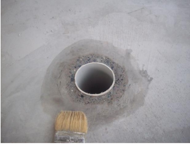
Figures 20H – 20I Apply the NOVITHOR Cementitious Parge so as to fill the trench and ensure it is flush against the exposed walls of the pipe penetration.
