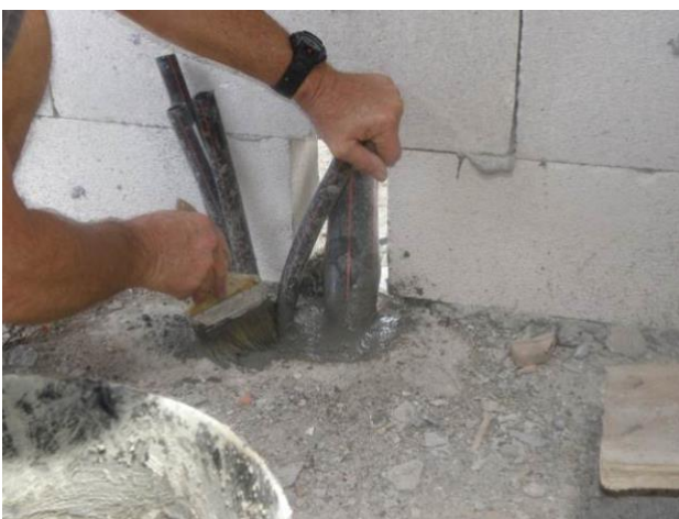
Figure 20B Apply NOVITHOR Cementitious Pargolite with soft bristled brush.
