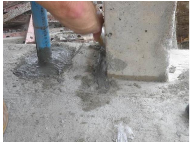
Figure 22 Ensure joint between pipe and concrete is fully covered. Cover cold joint between slab and RC column.
