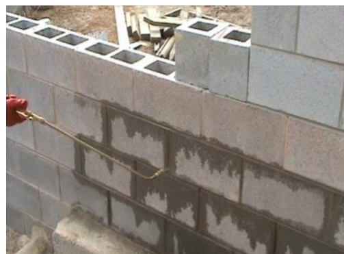
Figure 41 NOVITHOR Resin being applied to mortar joints in retaining wall.
