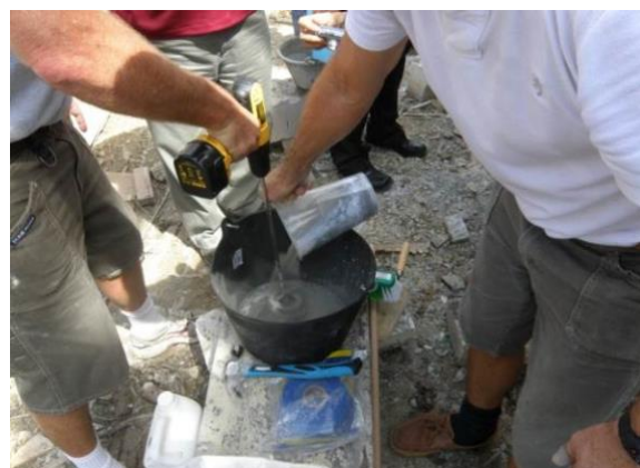
Figure 2 Mixing on site
