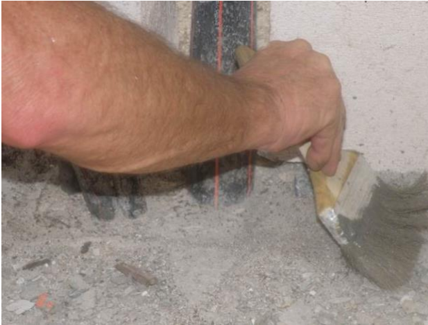
Figure 18 Remove loose dirt from around pipe and concrete.
