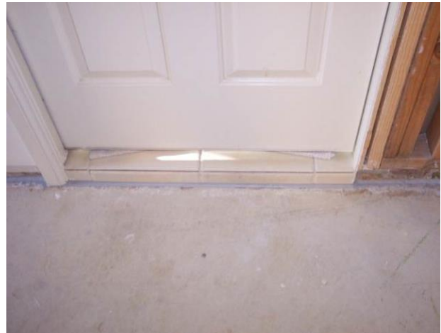
Figure 46 NOVITHOR Flexi-Gel between footing and garage floor in-fill slab.
