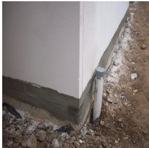
Figure 28 NOVITHOR Cementitious Parge applied over CSR Hebel and concrete slab edge.
