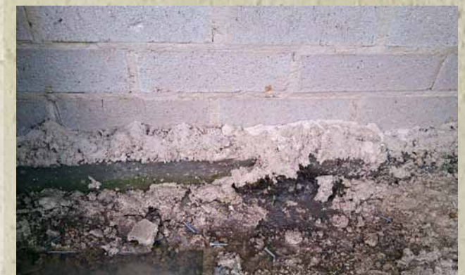
Excess mortar dropped during brick laying must be cleared from the base of the wall to allow installation.
