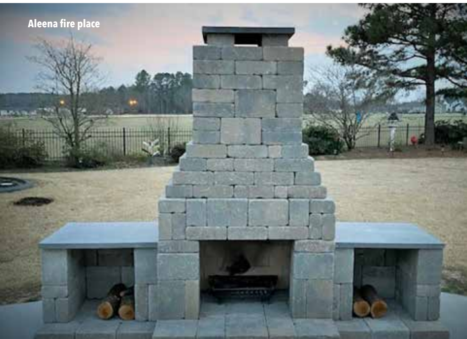
Custom Highland Fireplace, optional chimney cap
