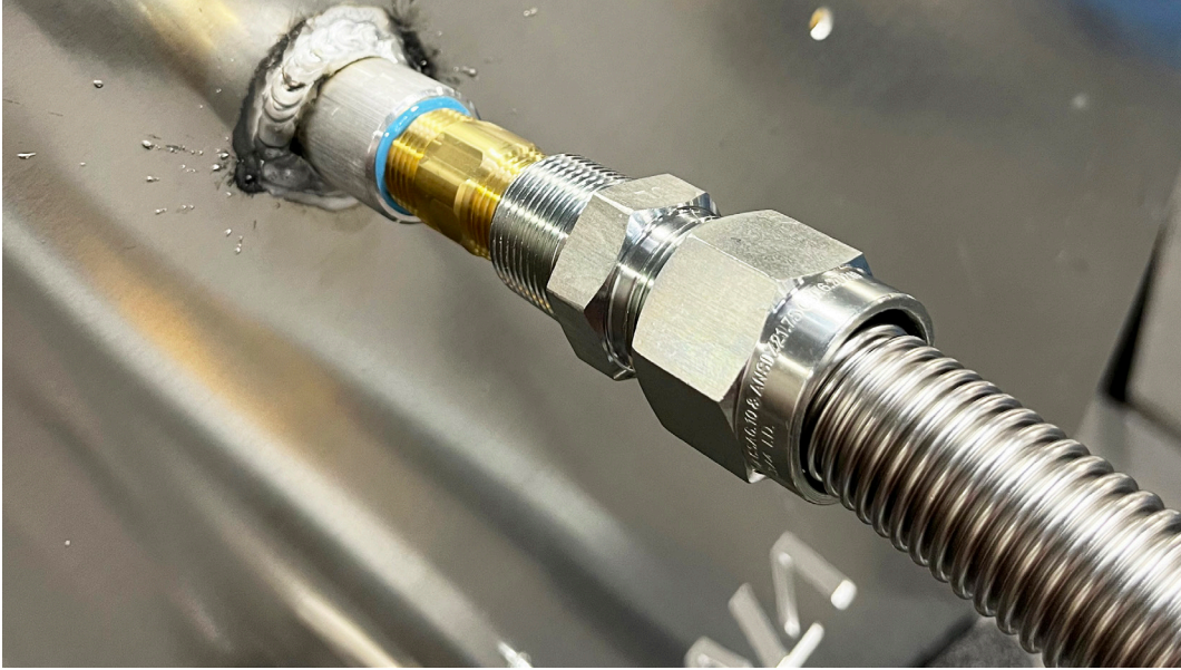
Photo 18: Connecting the Flex Line
