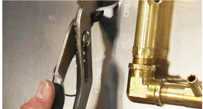
Photo 2: Breaking the Knockouts
