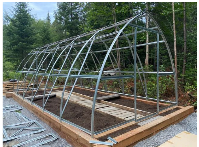
In the image: frame without legs, on a wooden base (the customer opted out of using them).
