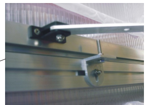
Window fixing with screw 4,2x16 to screw down
